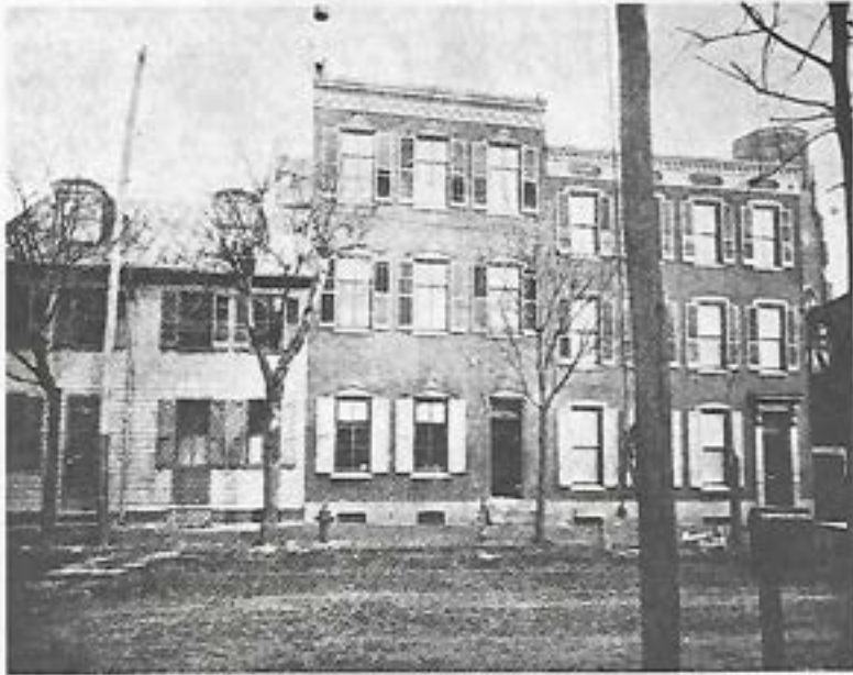
Rectory and Convent, Old Saint Lawrence Church Short Street
